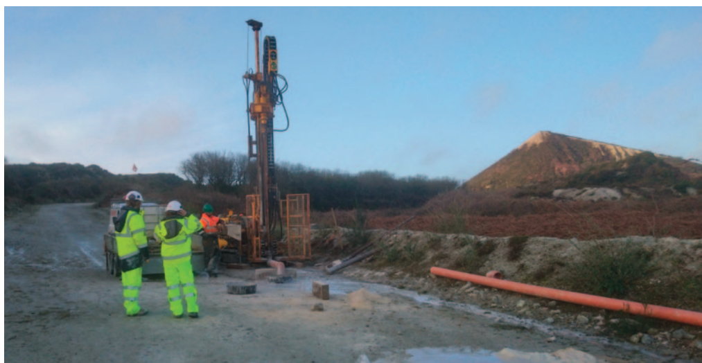
Hard rock Li drilling – Trelavour
